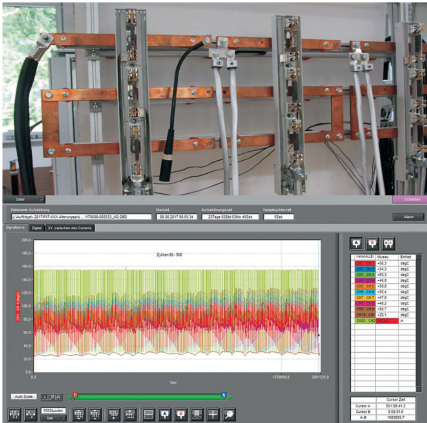
Photo 11. Testing of three disconnectors with V-type stacked terminals (with new spacer)
